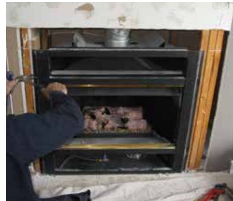
Remove unit from framing
